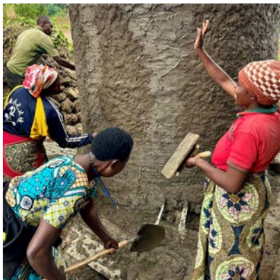
Left: Imbereheza members construct a household water tank; Right: a completed household water tank.
